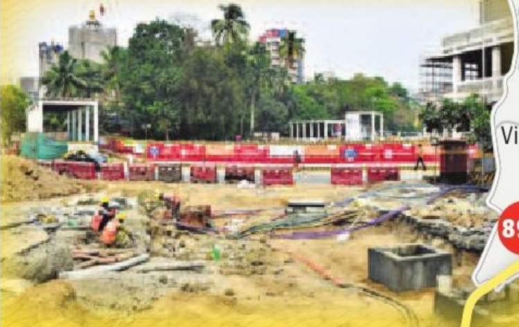
Construction work underway at Siddhivinyak station. BHUSHAN KOYANDE
