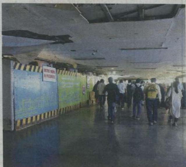
Barricades placed at old CSMT subway for the connector. PIC/ATUL KAMBLE
