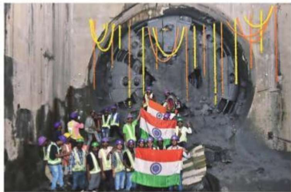
After final breakthrough on Wednesday. Photo courtesy: MMRCL
