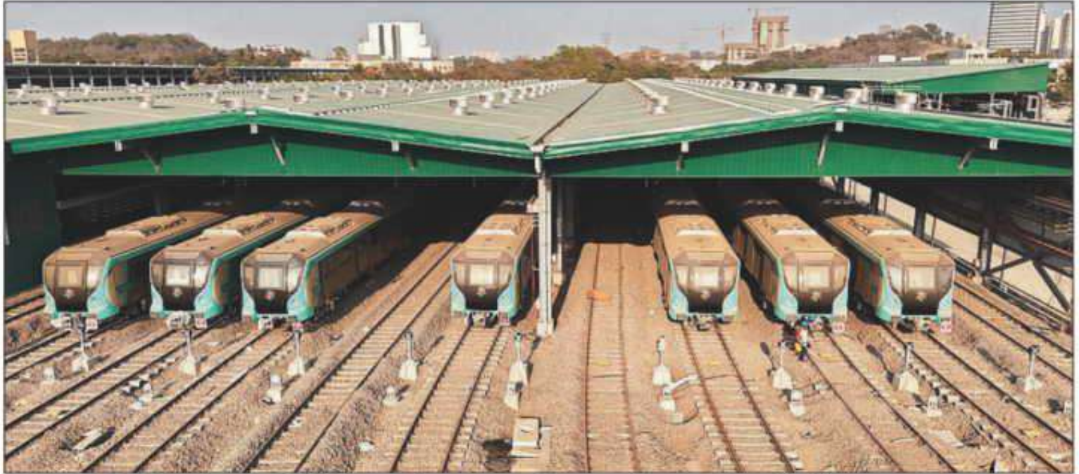
AAREY TO BKC: Only minor finishing works now remain, according to Metro officials
